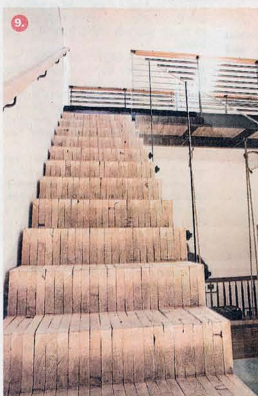
9. Salvaged lumber was glued together to form the butcher-block treads of the parlor staircase; chips and nail holes were left exposed. The railing is made of shower-door glass and industrial hardware.
